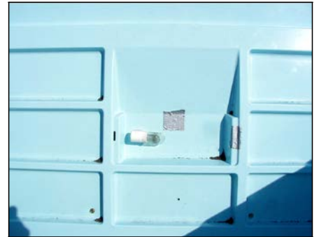
Mercury switch in a freezer
