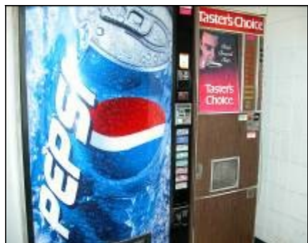
Prohibited: Ballast in fluorescent light of cooler unit
